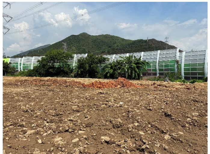
Photo 6: General view of the site
