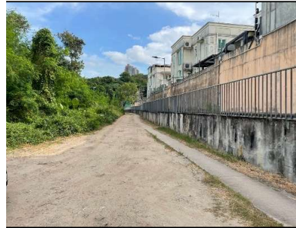
Existing Local Track Road to the Application Site
