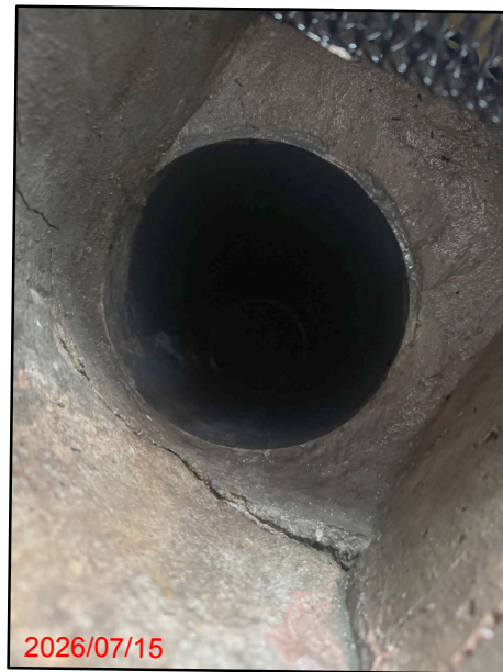
Existing 300 Dia. Drainage Pipe
