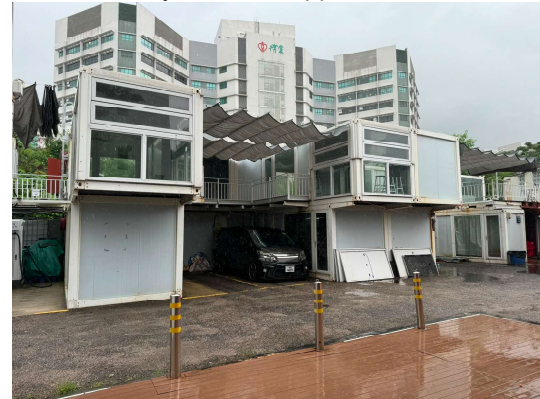
Photo 4: Block 2: Traffic Equipment Storage
