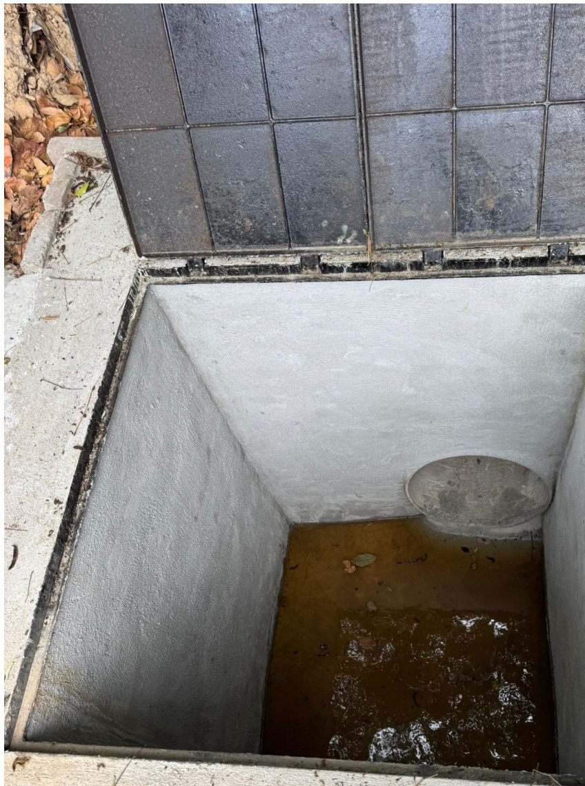
Photo No. V1 : Existing Catchpit and 525mm dia Pipe
