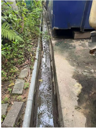
Photo no. A1
