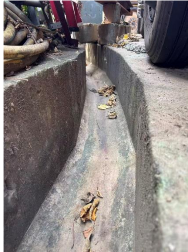
Photo no. A2
