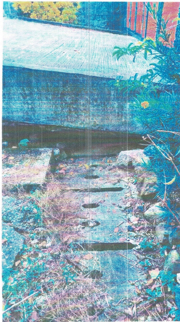
Photo 3 – Run-in Constructed under A/YL-SK/306 and U-Channel below
