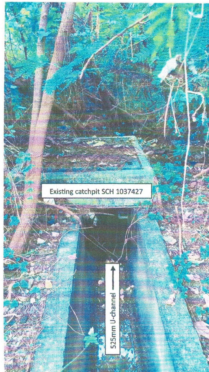
Photo 4 – Existing Catchpit and U-channel below Ko Sheung Road
