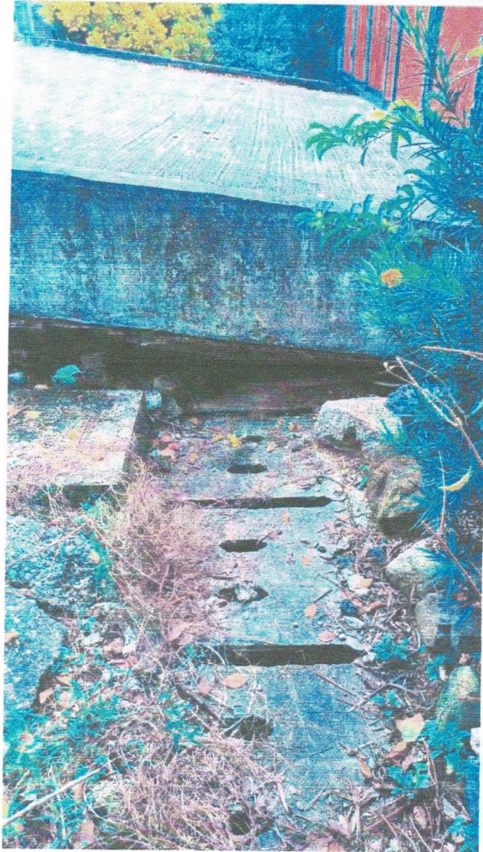
Photo 3 – Run-in Constructed under A/YL-SK/306 and U-Channel below
