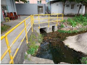
Plate 12 – Outfall of the existing 750mm U channel which receives discharges from the subject site at an existing watercourse
