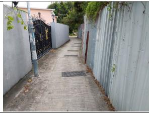
Plate 10 – Existing 750mm U channel receiving discharges from the subject site and running southwestward
