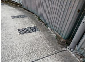
Plate 9 – Existing 750mm U channel receiving discharges from the subject site and running southwestward
