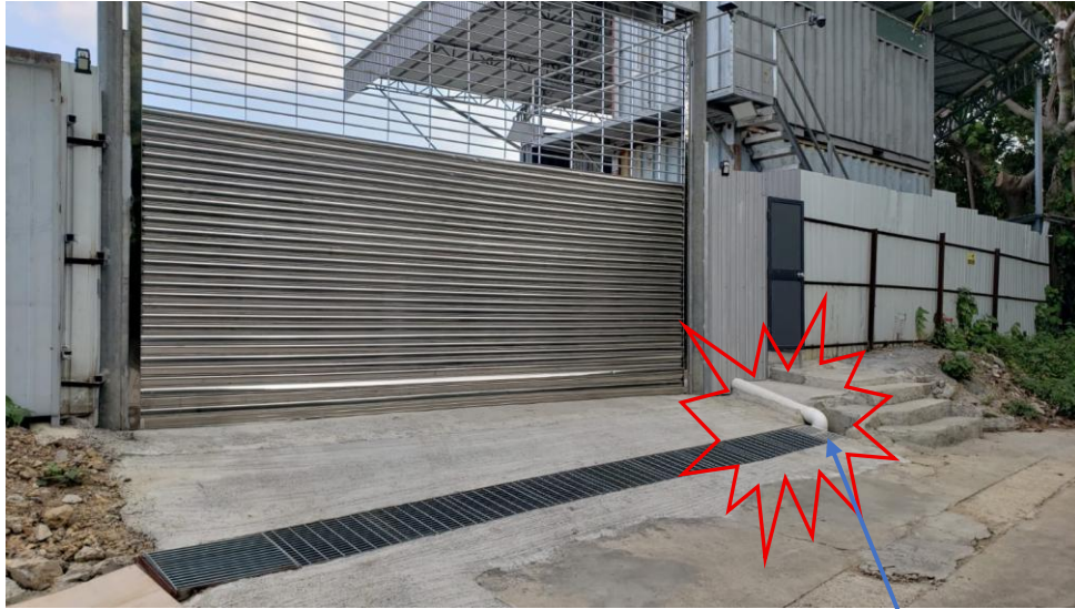
Photo 3: existing 300mm open channel The outlet non-standard catchpit was modified in May 2025
