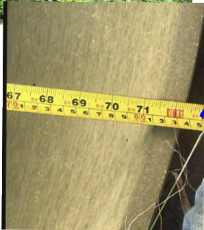
SITE PHOTO 7 EXISTING UNDERGROUND 1000mm dia. PIPE and Existing Stream
