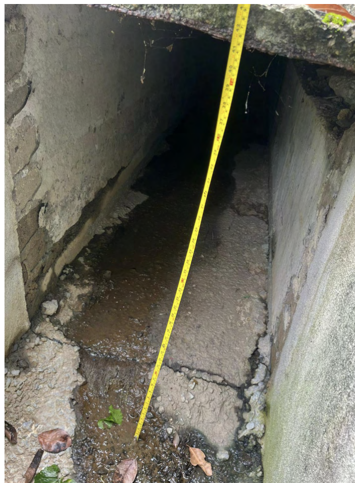
Dimension of 1000mm Box Culvert
