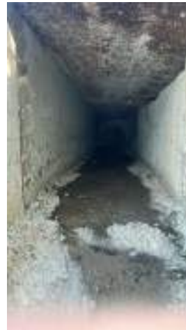
Site 5 Existing Underground 1000mm box culvet
