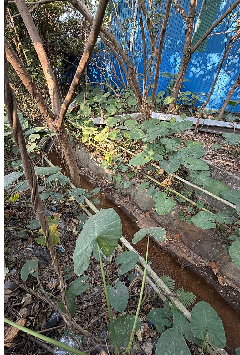
Photo 5 - Approximate 1mx1m open channel
