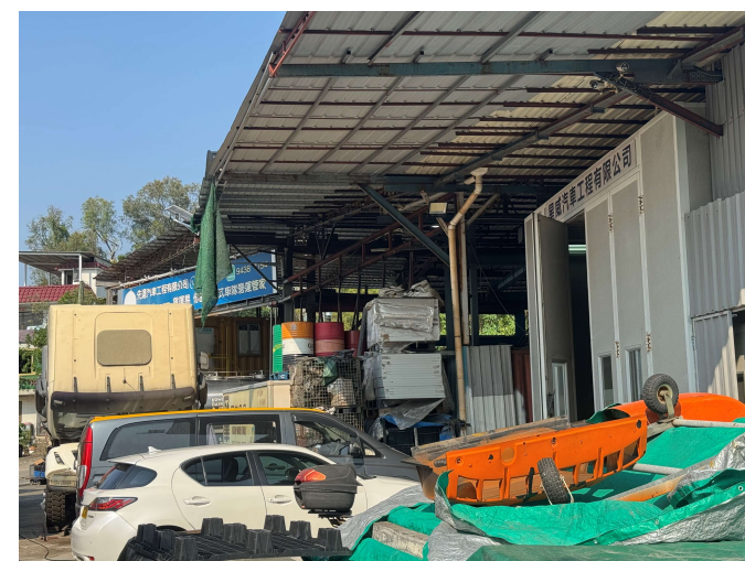
P-06 – Star Power Motor Engineering Ltd. (CR2)
