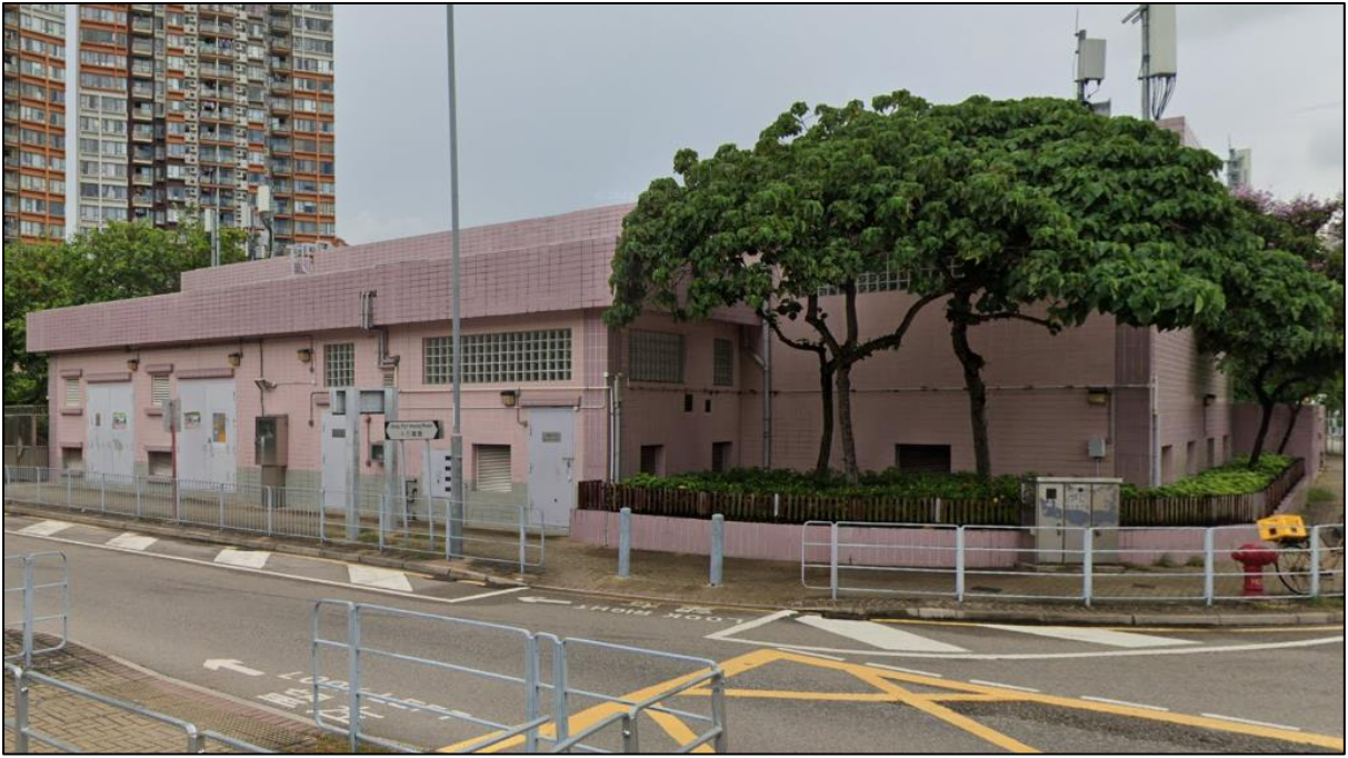
NS 01: Ma Tin Sewage Pumping Station
