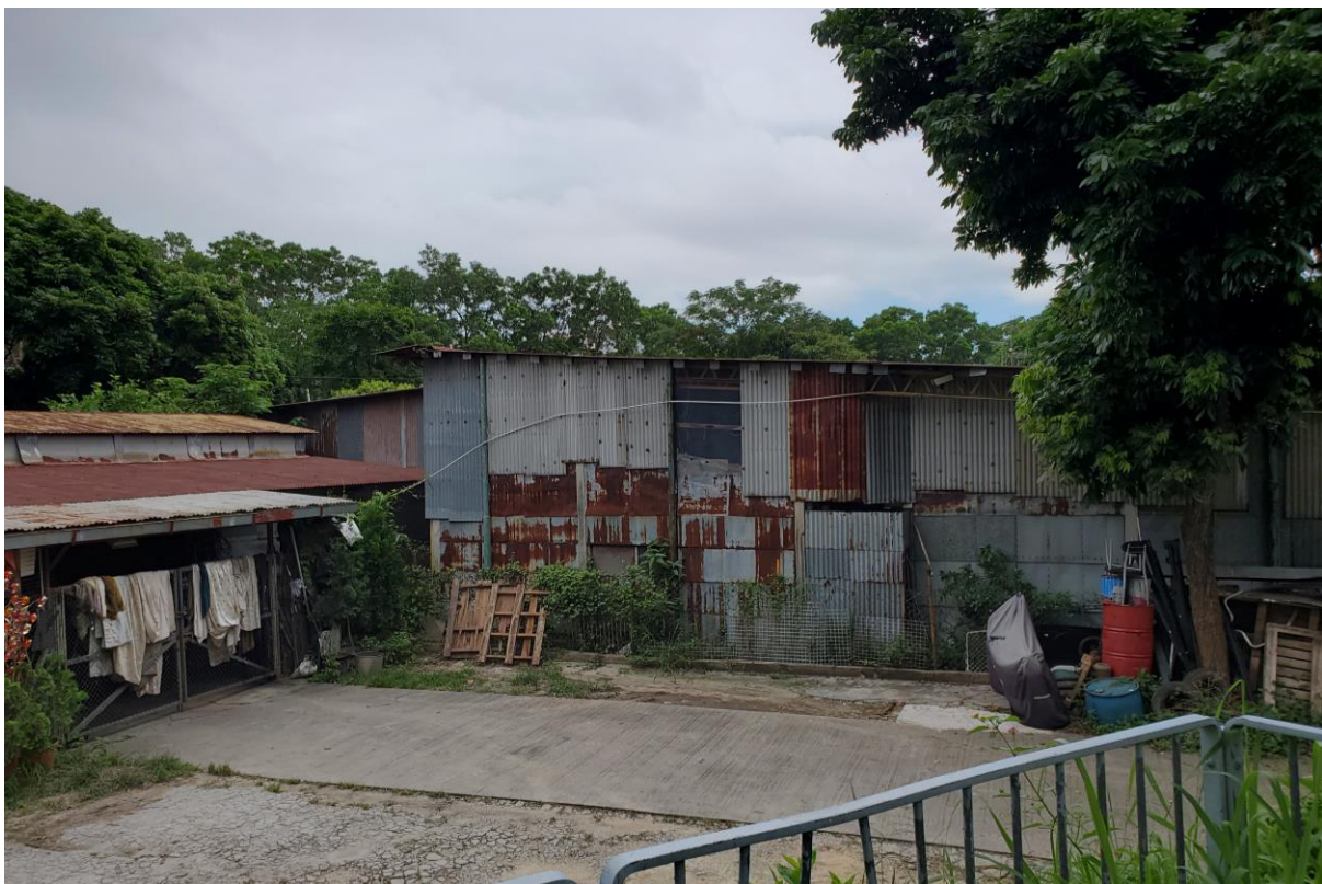
NS 08: Storage area along Lam Hi Roads
