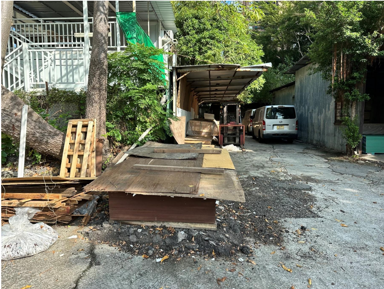
Appendix 5.4: Photo 1 – Temporary Structure within the Phase II Development Site
