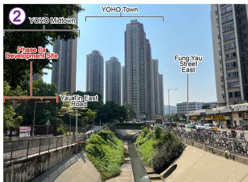
The nullah and residential developments near Application Site
