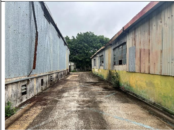
15. Concrete paved access road within the Application Site. Paint stains are observed with no crack.
