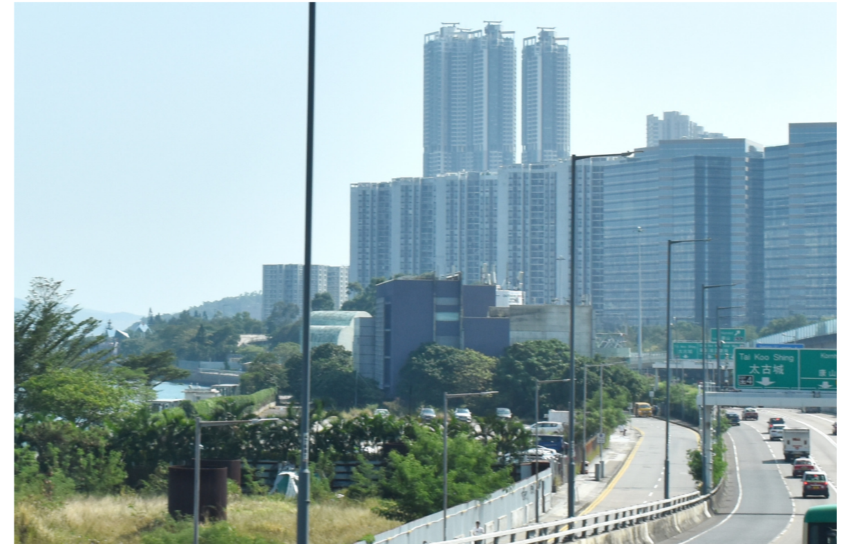
I Other visually detracting elements include the MTR Corporation ("MTRC") Quarry Bay Substation and EHT Quarry Bay Ventilation Building
