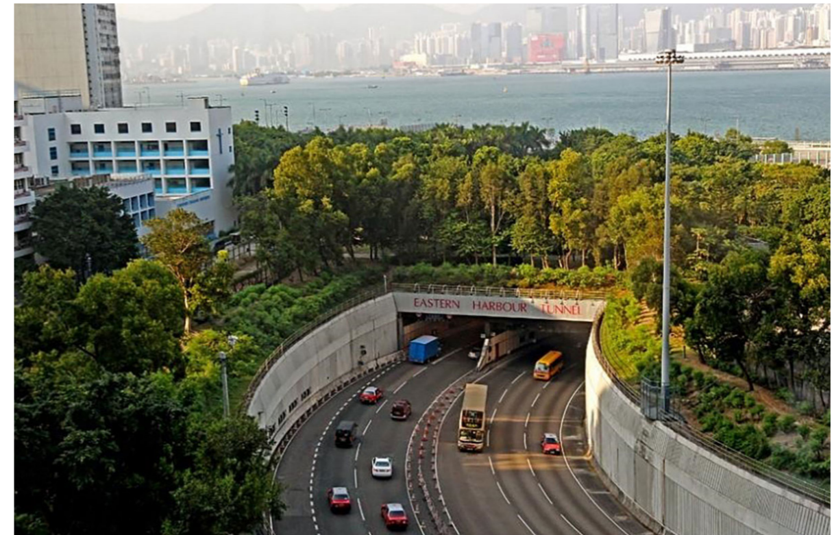
K Major infrastructure including the approach roads and tunnel portal for the Eastern Harbour Crossing
