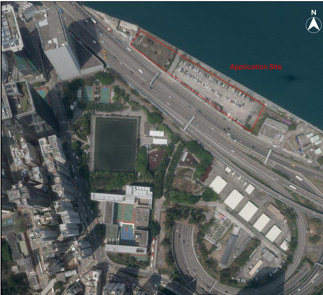
Figure D-8 Aerial Photo in March 2024
