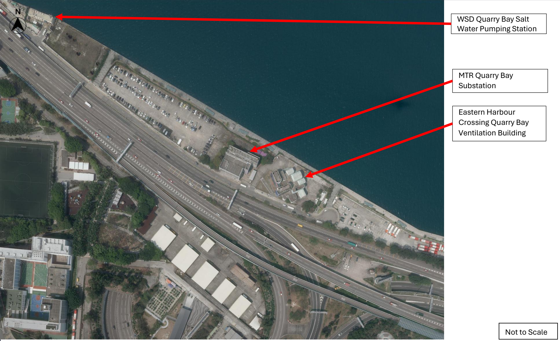
Figure 3-2: Identified Fixed Noise Sources at the Vicinity of the Site
