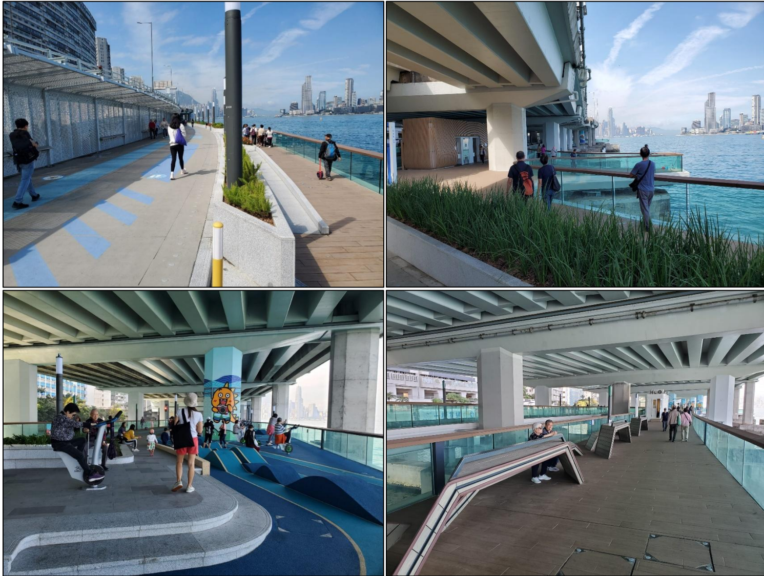
Figure 8: Western Section of the IEC Boardwalk is open for public access and is a spectacular new viewing route along the waterfront
