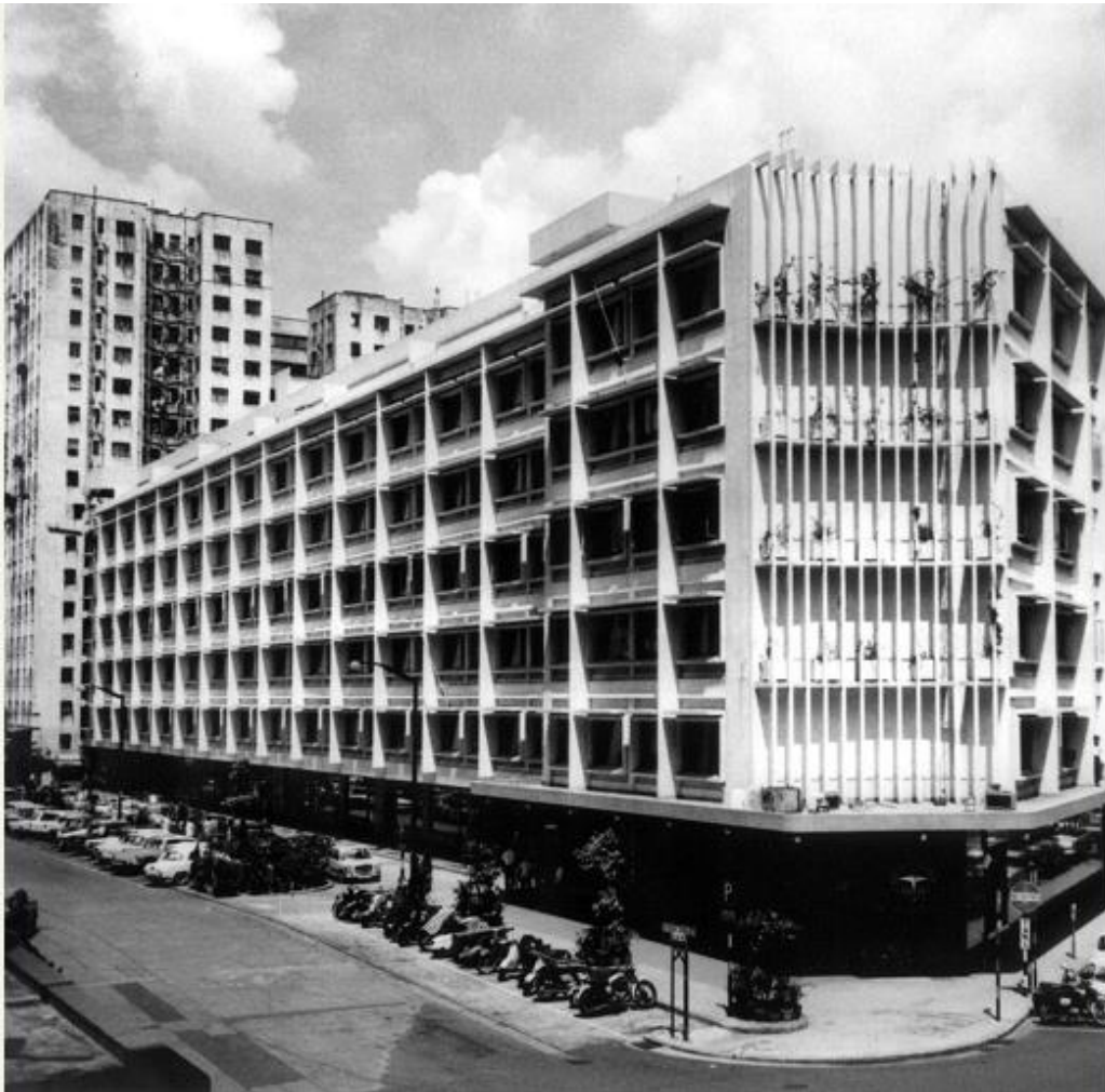
Photograph 4: The construction of the six-storey Lee Gardens commercial building was completed in the late 1960s. The photograph of the completed commercial building clearly shows the presence of both the drop-off and the adjoining car park along Hysan Avenue.
