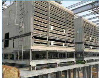
Hongkong-Zhuhai-Macau Bridge China FWS-700-37-GI x 7
