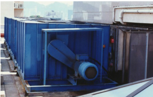
Oily fume treatment system on the roof
