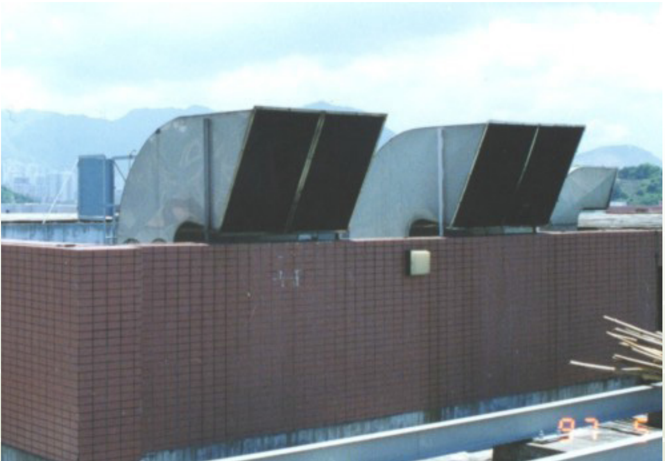
An example of good practice, extending kitchen exhausts to rooftop
