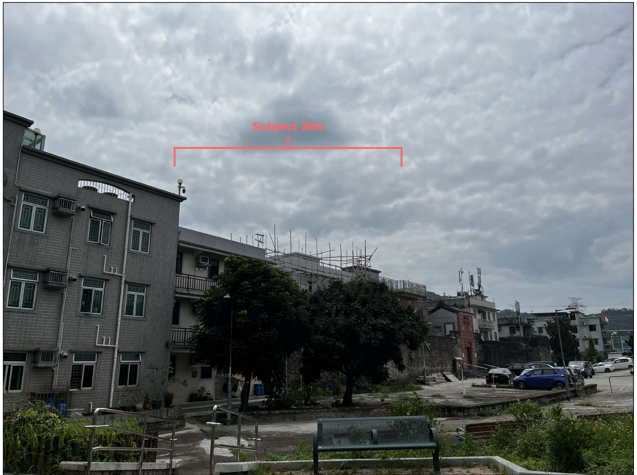
Existing condition (Scheme A)
