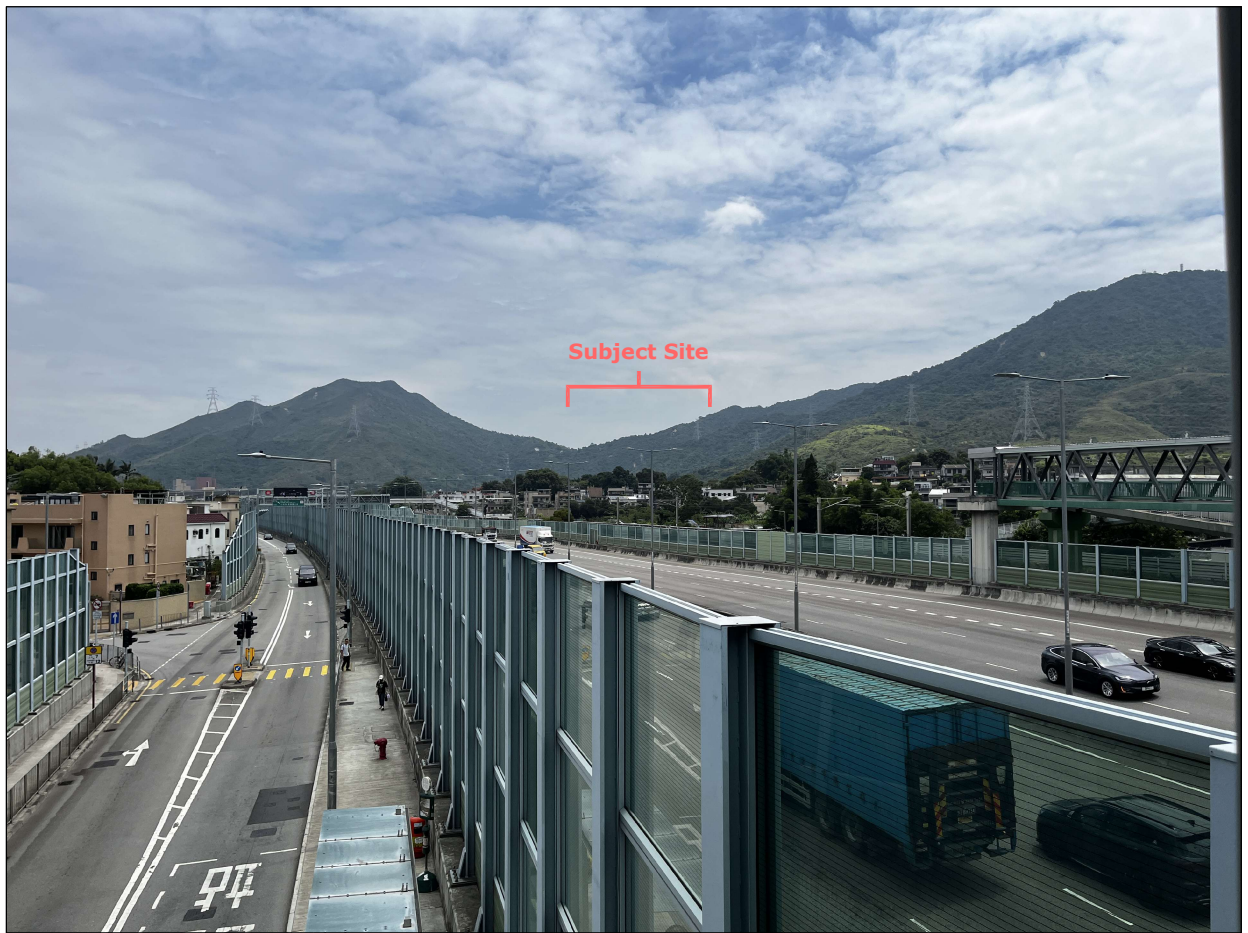
Existing condition (Scheme A)
