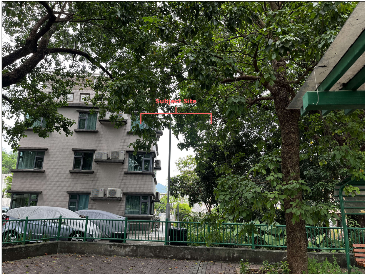
Existing condition (Scheme A)
