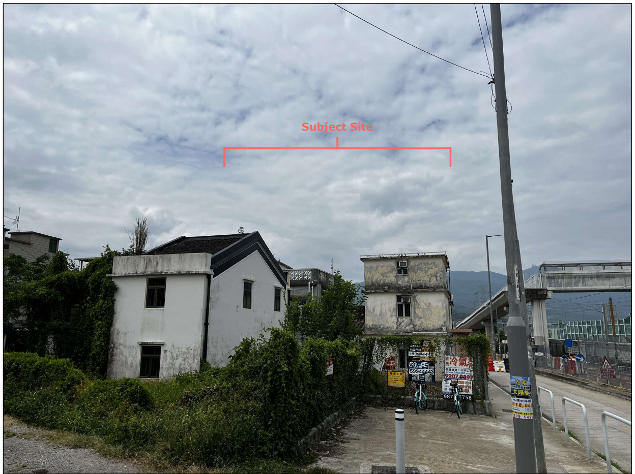
Existing condition (Scheme A)
