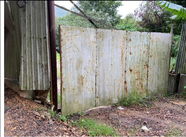
Photo 1: The site cannot be accessed.
