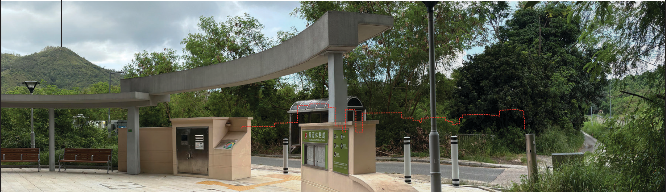
Vantage Point 08: View looking north west towards the site from Cheung Lek Sitting-out Area (Proposed Scheme)
