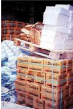
Figure 3.12 Improper stacking of blocks
