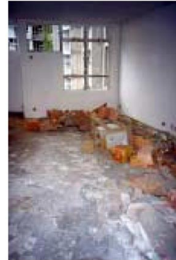
Figure 3.14 Cutting waste of tiles
