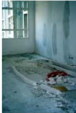
Figure 3.10 Cutting waste of dry wall
