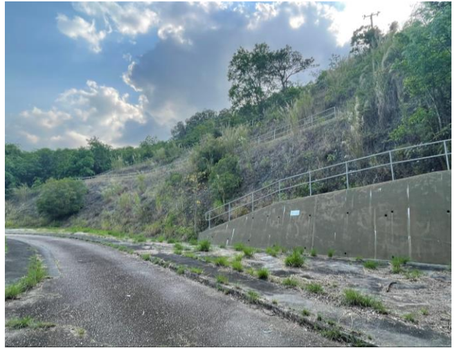
③ Current Access to River Ganges Pumping Station
