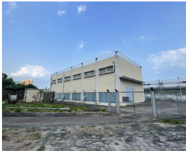
① River Ganges Pumping Station
