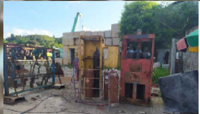
acetylene cylinders found (improper storage)
