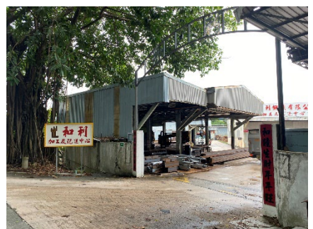
7 Existing rural workshop
