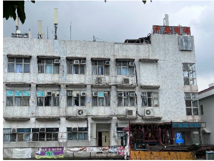
3 Ping Che Commercial Centre and Ping Che Nursing Home Limited
