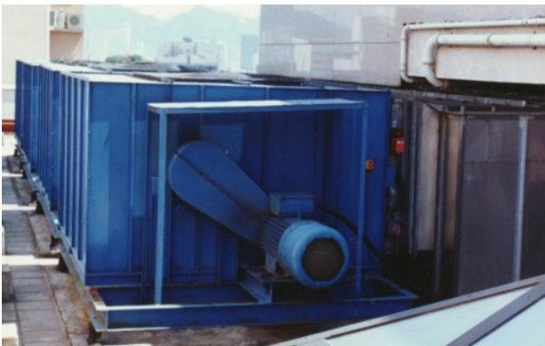
Oily fume treatment system on the roof
