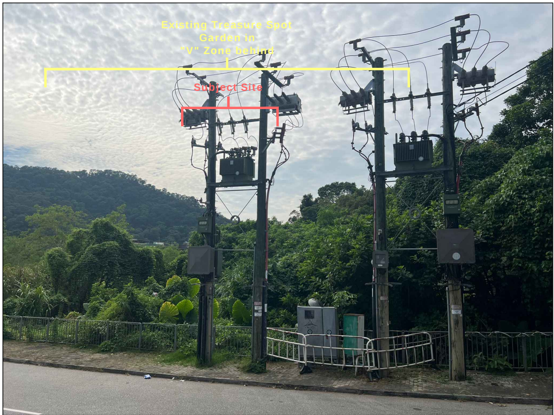
Existing condition (Scheme A)
