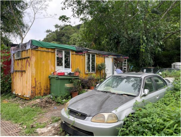
④ Temporary structures
