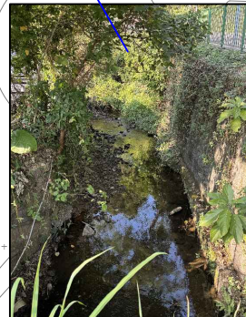
1. Nullah at the entrance of the site
