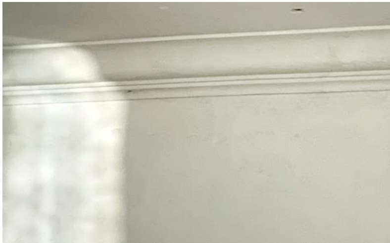
B4.3.31 – Ceiling corner crown moulding at Main Building.
