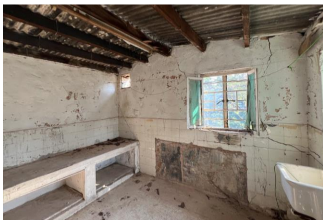
B5.4.2 – The later added kitchen on the roof, Main Building.
