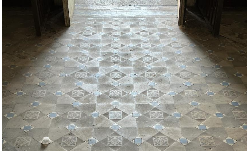
B4.3.19 – Ornate tile flooring at the entrance hallway, Main Building.
