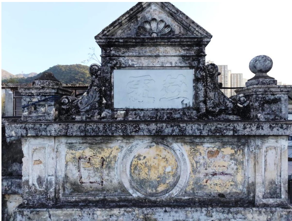
B7.3.20 Roof balustrade wall with pediment in 2025 Dec. (Source: Nam)
