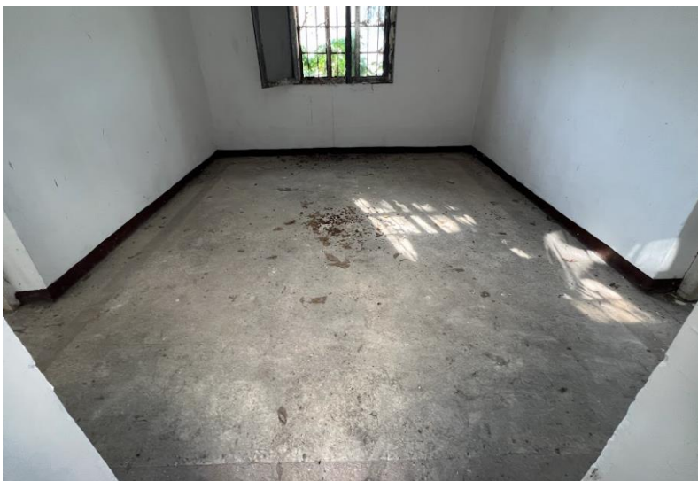
B4.3.24 – Terrazzo flooring with vermillion border, Sub Building.
