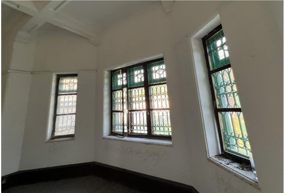
B4.3.11 – Windows at the G/F living room, Main Building.
