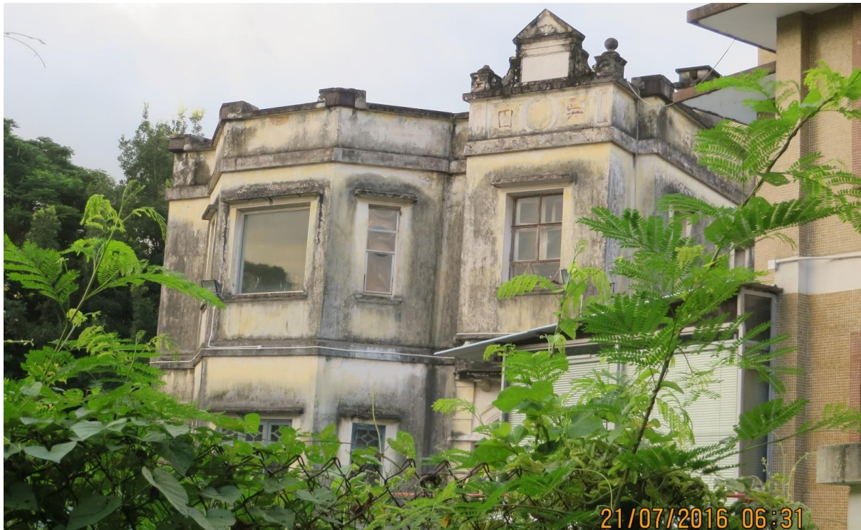
B7.3.14 Roof balustrade wall with pediment in 2016.
