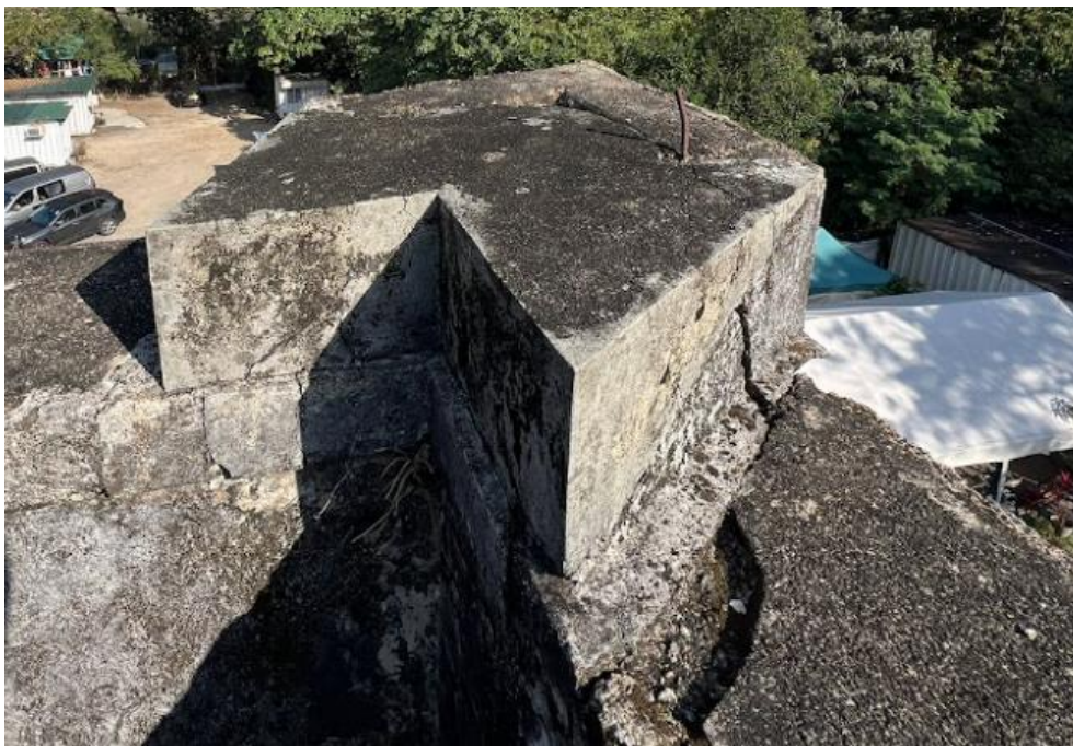
B4.3.6 – Roof crenellation features as observed from roof level, Main Building.
