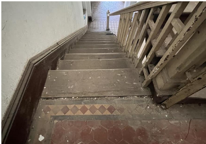
B4.3.23 – Teak flooring at the staircase at Main Building.
