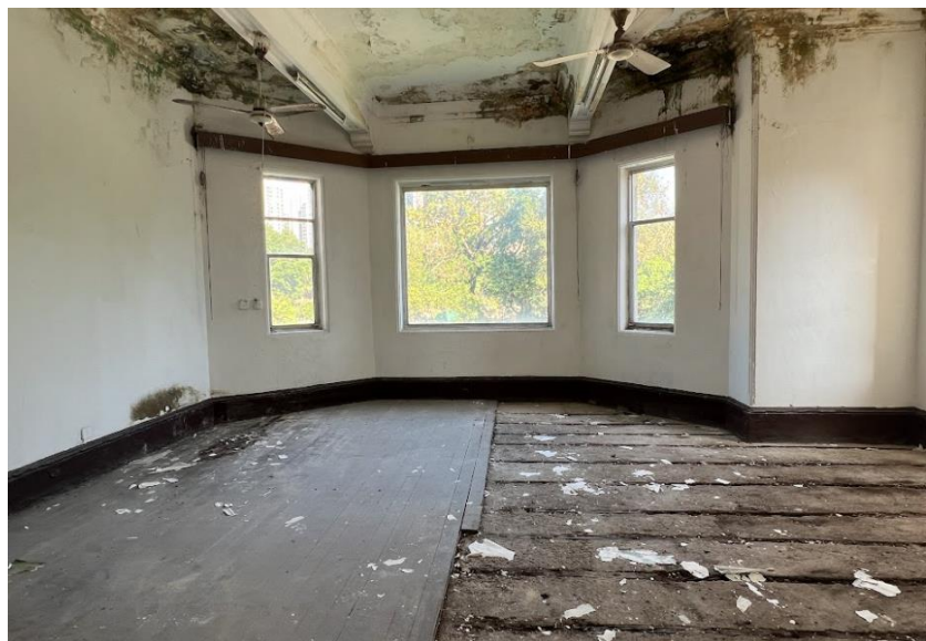
B4.3.21 – Teak flooring at 1/F dining room, Main Building.
