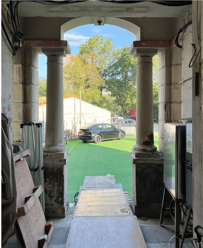
B4.3.2 – Entrance arch porch, Main Building.
