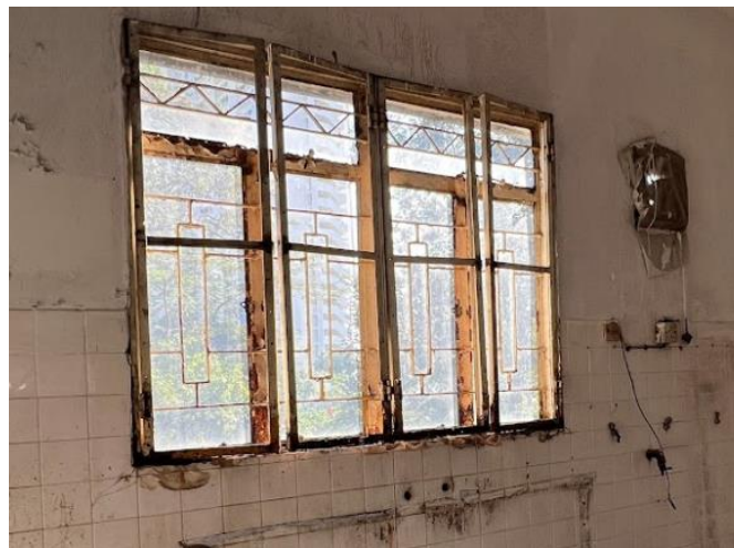
B5.3.5 – The window frames and ironmongery of the 1/F kitchen, Main Building.
