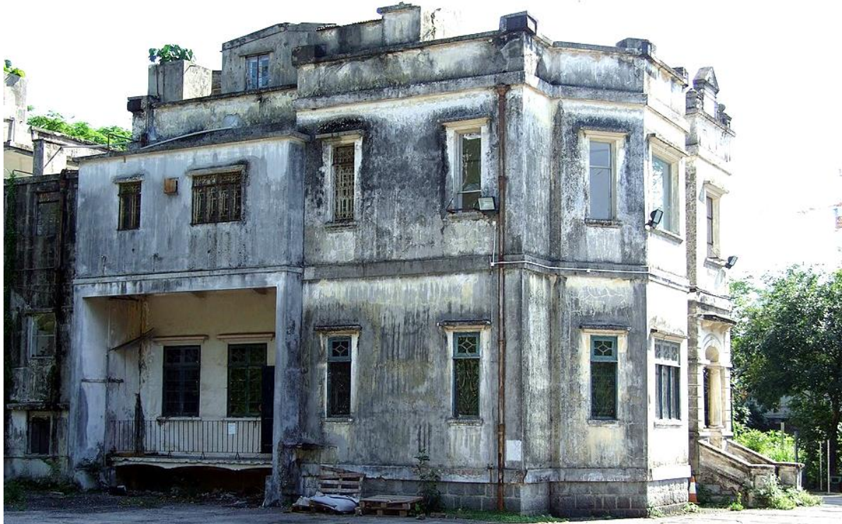
B7.3.6 Side (east) elevations in 2010.
