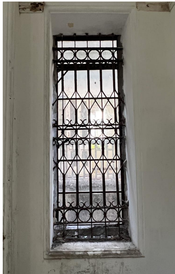
B4.3.9 & 10 – Metal grilles are installed at sidelights of the G/F main entrance, and other G/F windows, Main Building.
