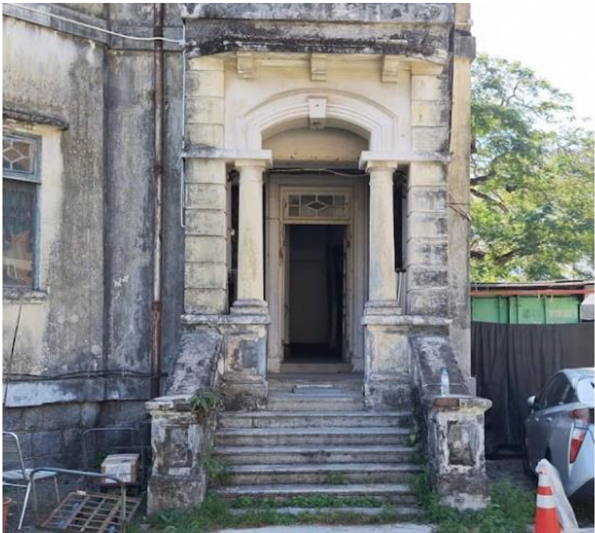
B4.3.1 – Entrance arch porch, Main Building.
