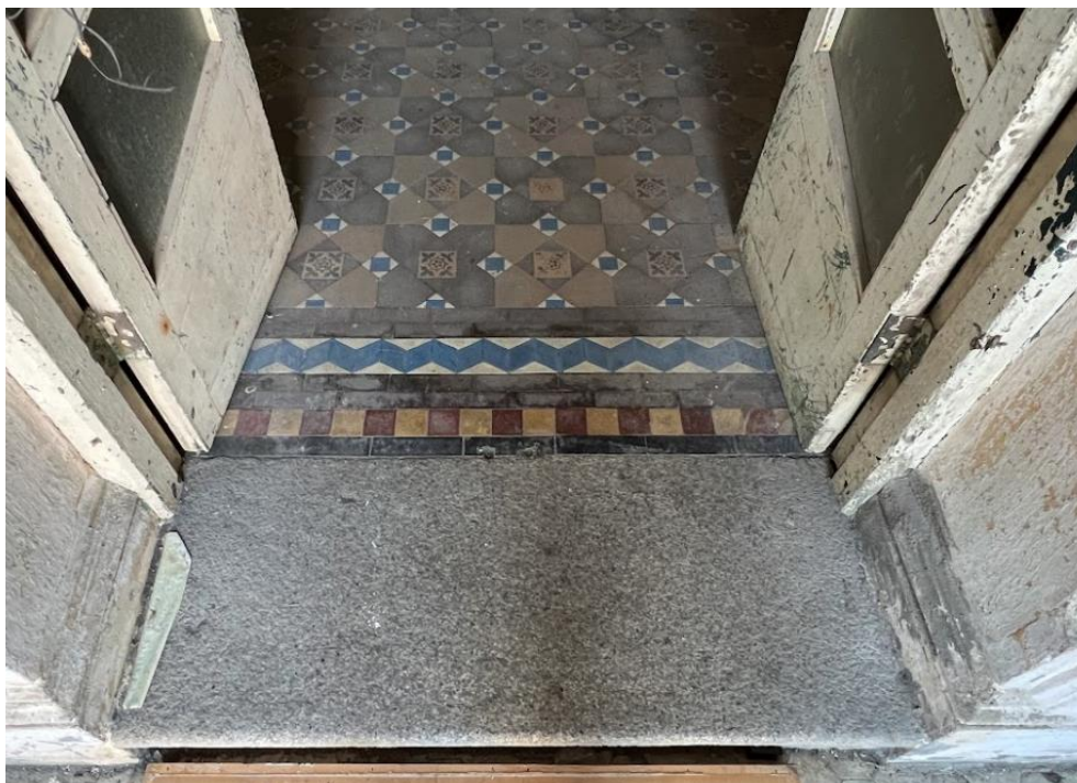
B4.3.18 – G/F entrance granite threshold ornate tile flooring, Main Building.
