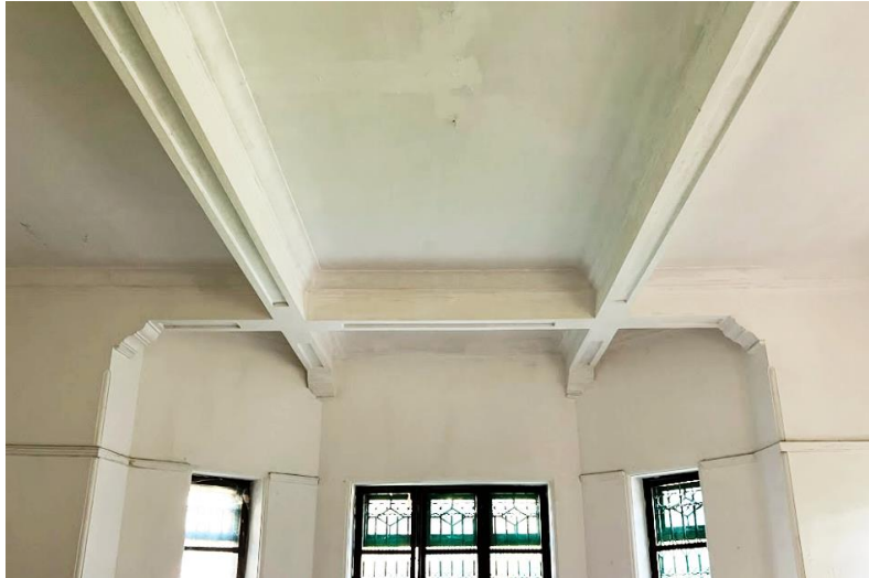
B4.1.4 – Structure with reinforced concrete structural beams at Main Building.
