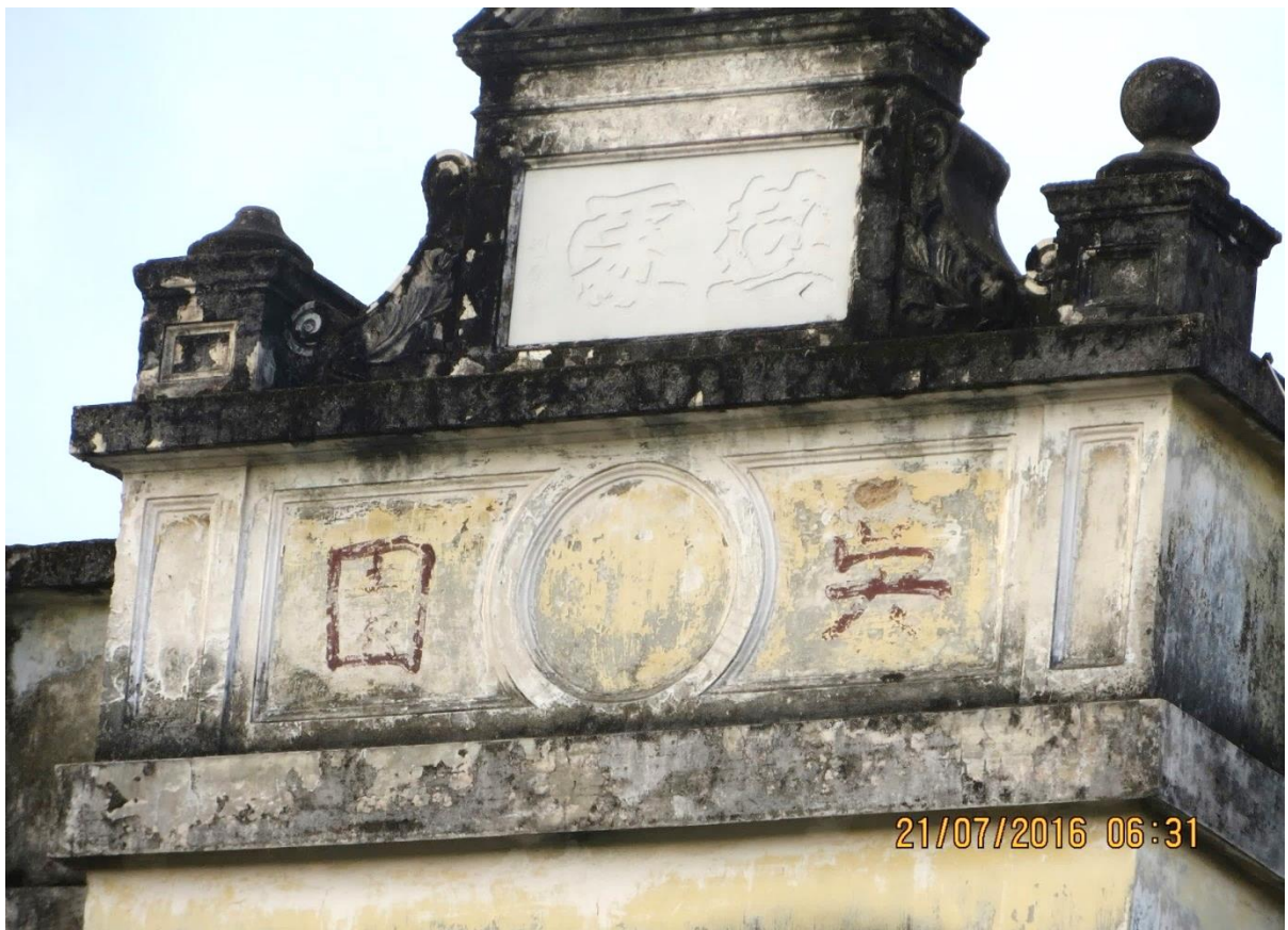
B7.3.15 Roof balustrade wall with pediment in 2016.
