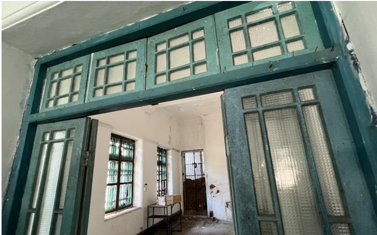
B4.3.16 – G/F partitioning doors, Main Building.
