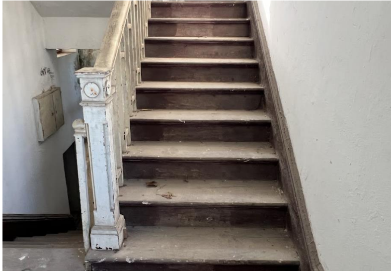
B4.3.27 – Teak flooring at the interior staircase at Main Building.
