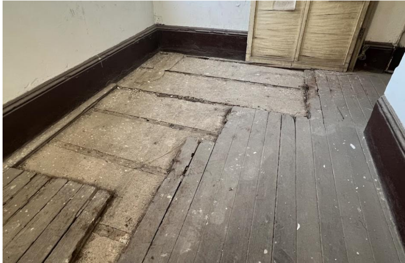
B4.3.22 – Teak flooring at a room on the 1/F, Main Building.
