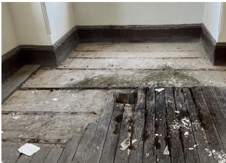
B4.1.6 – Slabs composed of reinforced concrete structural slab blocks inserted with timber strips.
