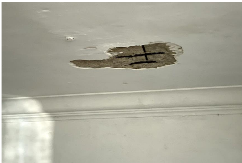
B4.1.5 – Structure with reinforced concrete slabs at Main Building.
