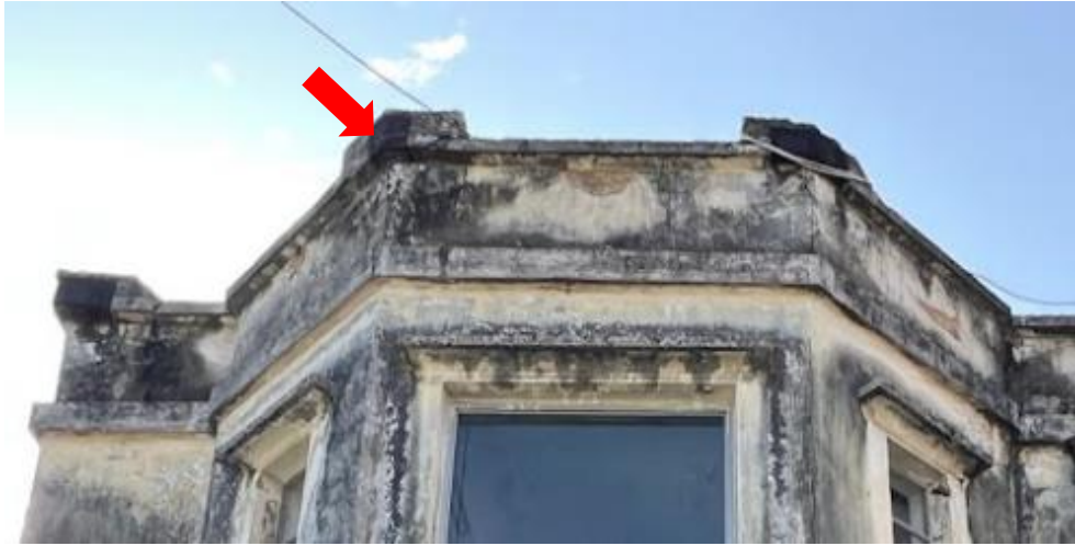
B4.3.5 – Roof crenellation features as observed from street level, Main Building.
