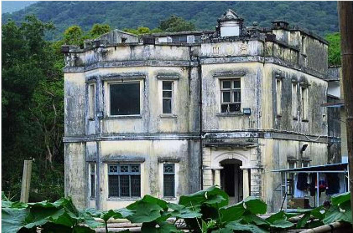
B7.3.11 Front (north) and side (west) elevations in 2012. (Photo by Tere Wong. Source: https://blog.terewong.com/archives/7434 )
