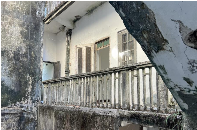
B4.3.28 – Concrete balustrades along the corridors at the Sub Building.
