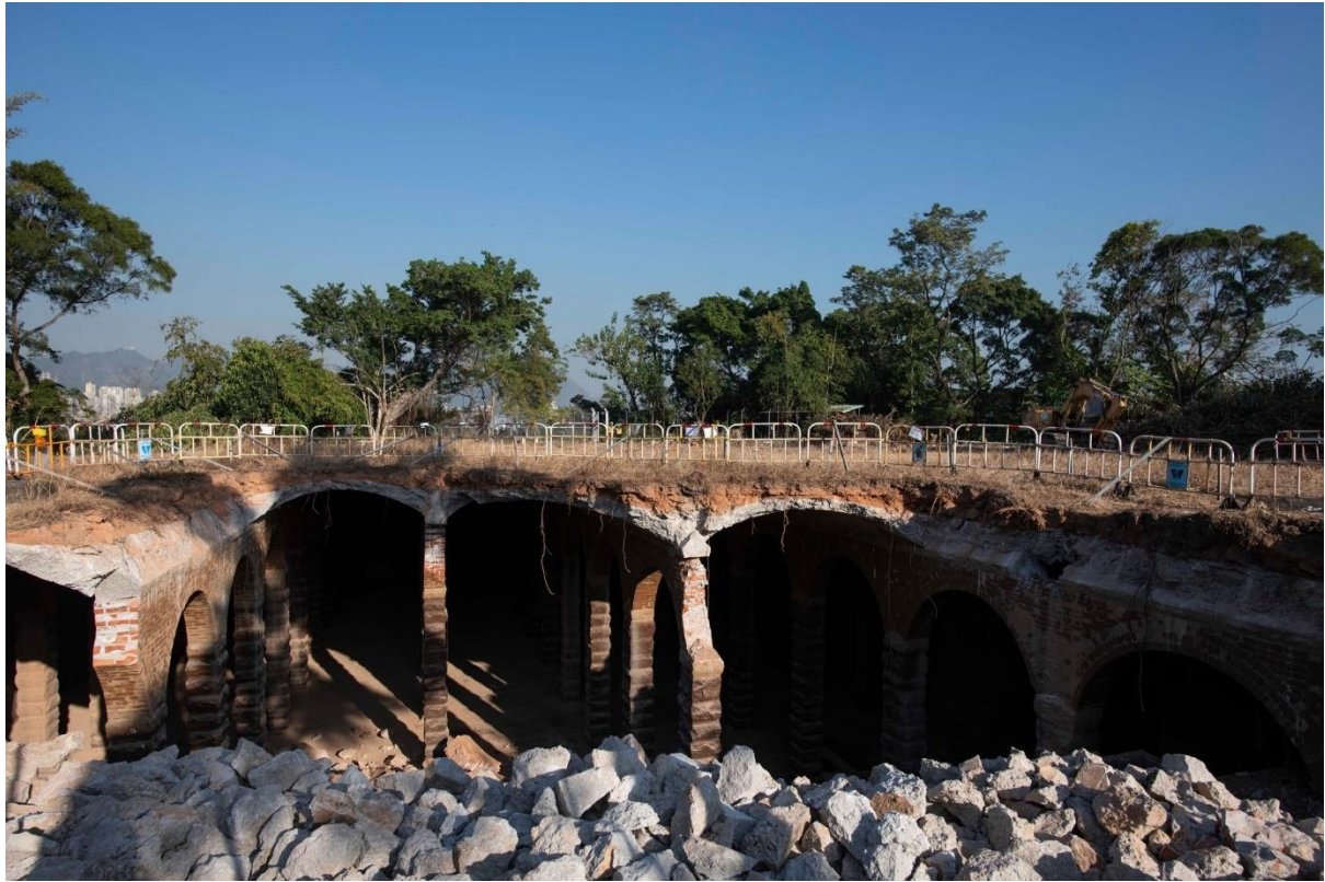
B.3.2 – Ex-Sham Shui Po Reserve Reservoir was constructed by Tung Shing Construction Co.. (Source: HKTkww)
