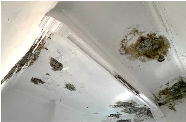
B4.3.30 – Ceiling corner crown moulding, Main Building
