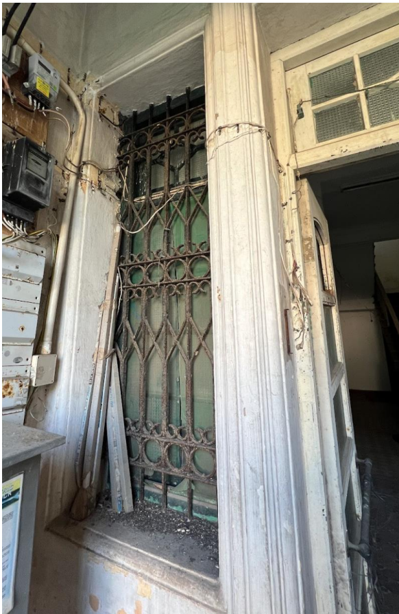
B4.3.9 & 10 – Metal grilles are installed at sidelights of the G/F main entrance, and other G/F windows, Main Building.
