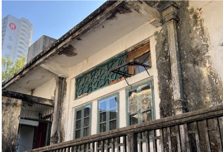
B4.3.13 – Fanlights with timber carving, Sub Building.
