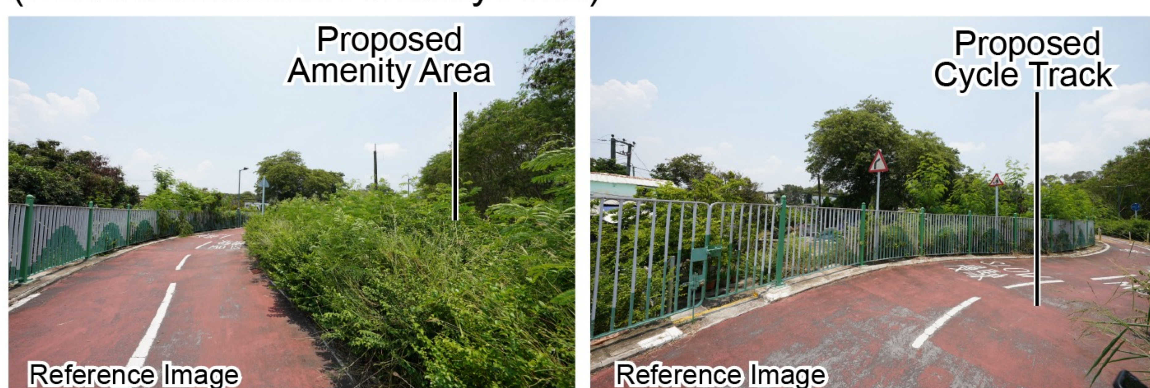
Under CEDD's Project (with inaccessible Amenity Area)
