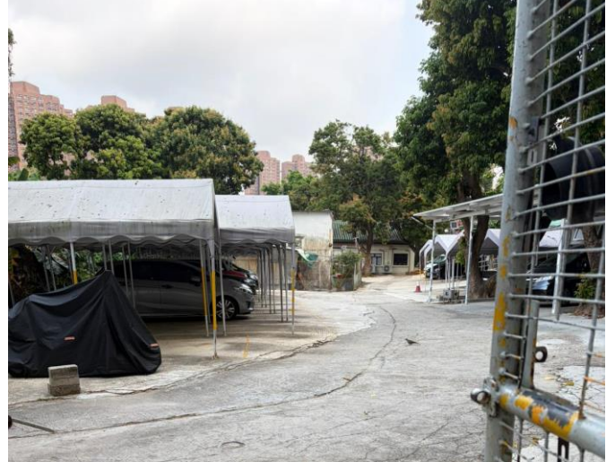
Temporary Structures to the northeast of the Site (P16)
