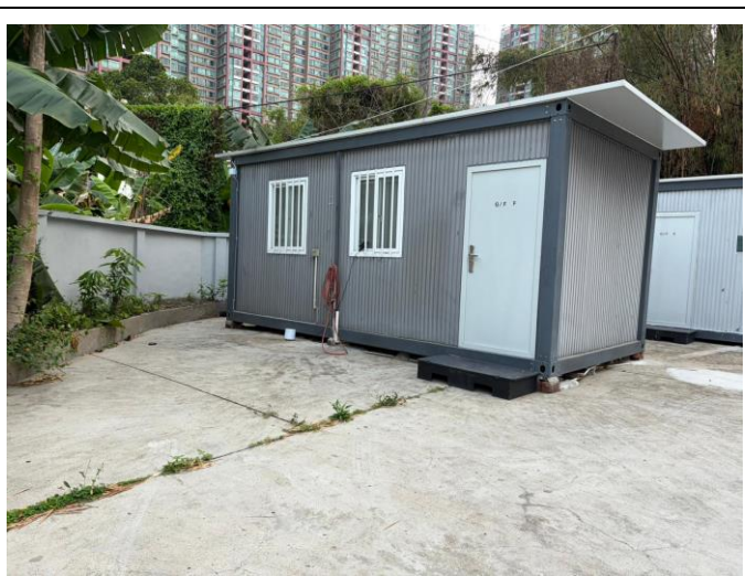
Photographic Record: (P06) Enclosed structure is located in the Site for residential uses.
