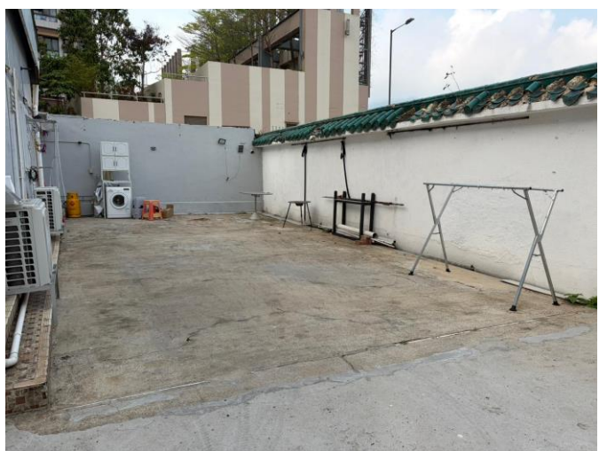
Photographic Record: (P08) The site is fully covered by concrete slab, and the ground is observed to be in good condition.
