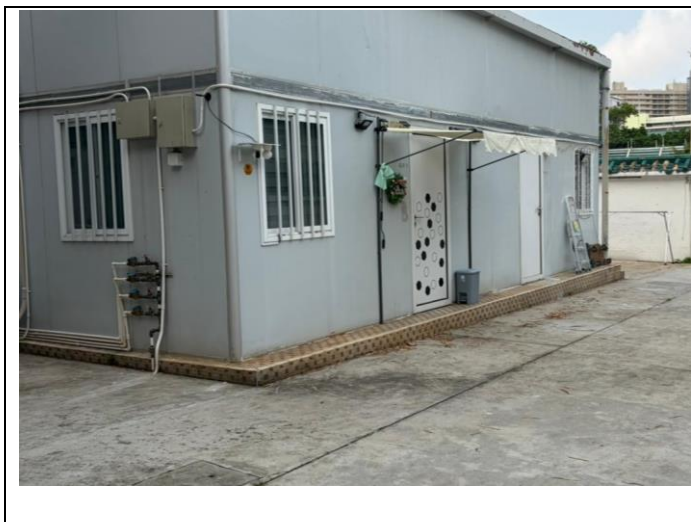
Photographic Record: (P05) Enclosed structure is located in the Site for residential uses.
