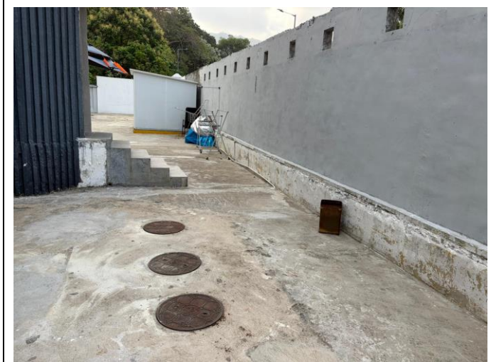
Photographic Record: (P07) The site is fully covered by concrete slab, and the ground is observed to be in good condition.
