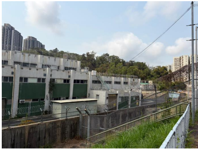
Tuen Mun Water Treatment Works (P01)
