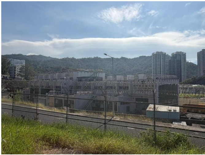
Tuen Mun Water Treatment Works (P01)
