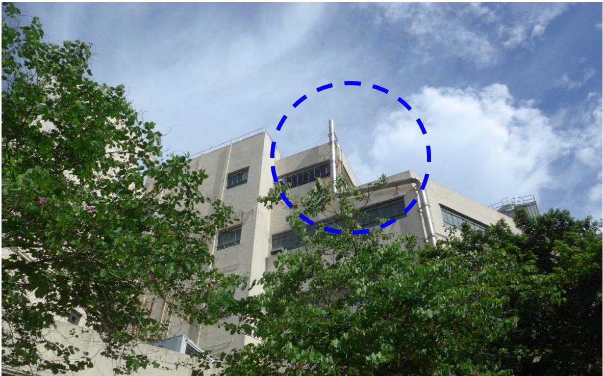
Plate 6: The chimney at GMP Centre (Source ID: GMCH01)
