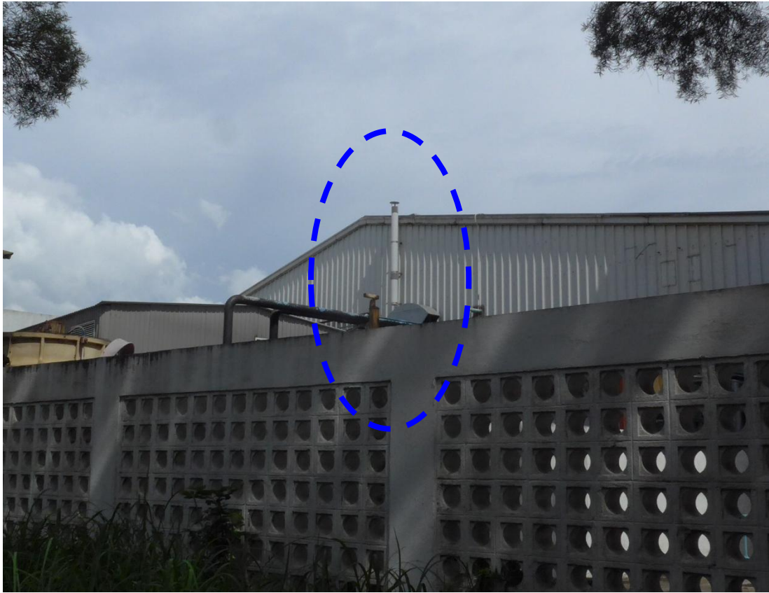
Plate 11: The chimney at Mass Lam int'l Ltd. (Source ID: MACH01)
