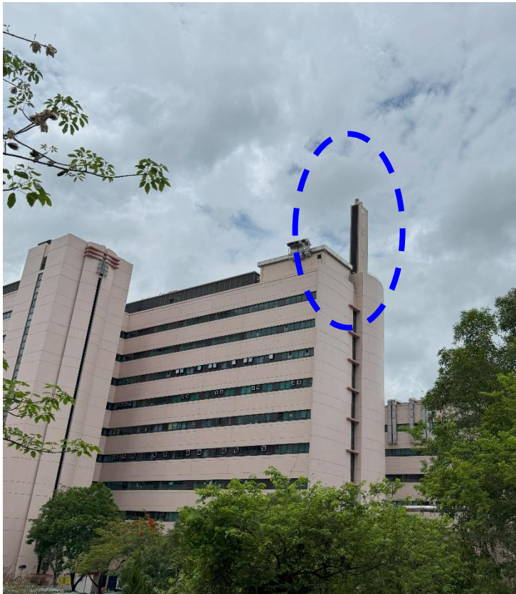
Plate 13: Towngas boilers at Alice Ho Miu Ling Nethersole Hospital (Source ID: NH01-02)
