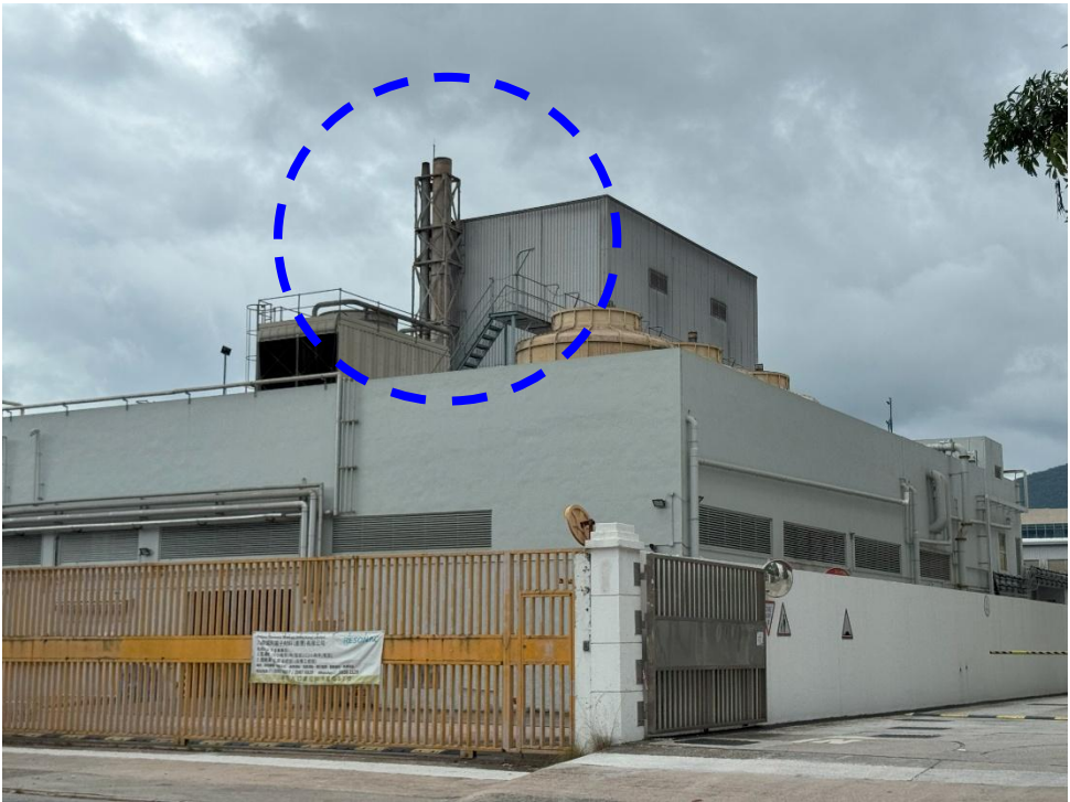
Plate 5: The chimney at Hitachi Chemical Electronic Materials (Hong Kong) Ltd. (Source IDs: HICH01 and HICH02)
