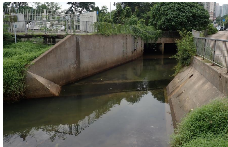
Channelised watercourse (Fung Yuen Stream)
