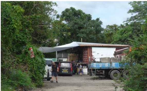
Electric screwdriver was observed. All operations were taken place under the cover
