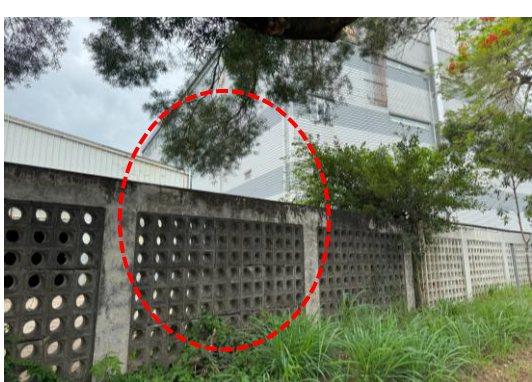
Cooling tower was removed
