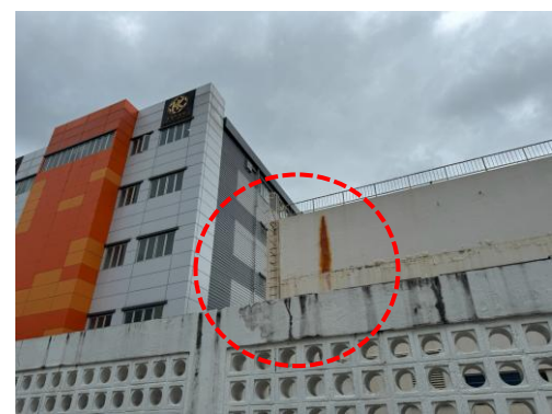
Cooling towers were removed
