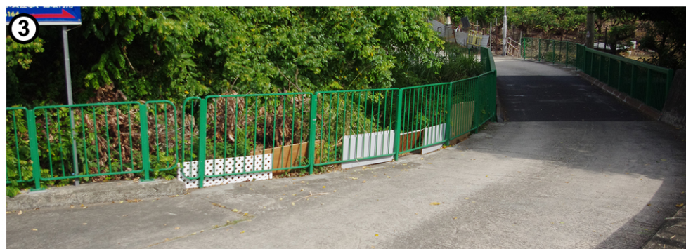
Existing entrance of local access in Site 2 connecting the local village / rural settlements with Kam Tin Road
