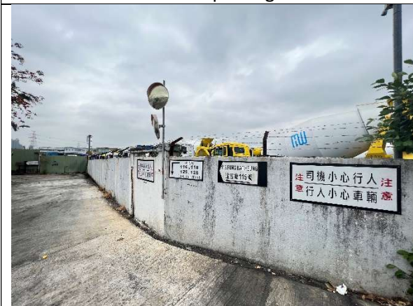
Photo 11: Boundary wall of the open car park
