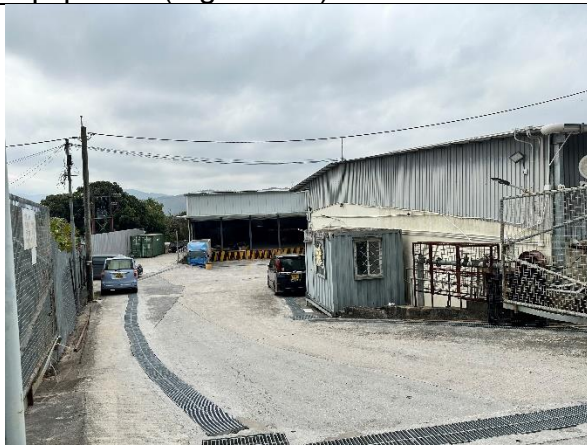
3. Warehouse with loading and unloading area, no noisy activity or equipment (e.g. forklift) is observed.
