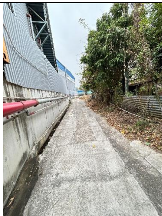
Photo 11 A gully surrounds the warehouse and the logistics company.
