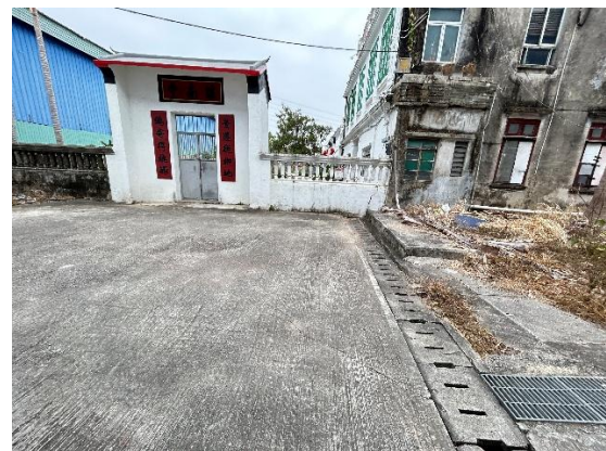
Photo 12 A gully for Shum Residence is connected to gully for warehouse and logistic company.
