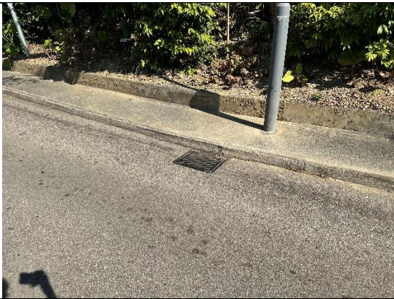
Photo 15 A road gully is located along the road to the north of the Application Site.
