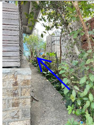
Photo 4 A gully is connected to the warehouses located on the north side of Fung Kat Heung Road.
