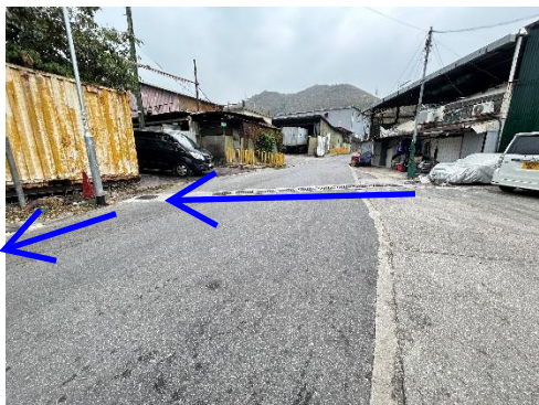
Photo 5 A road gully crosses Fung Kat Heung Road and is connected to the drainage channel along the north side of Fung Kat Heung Road.
