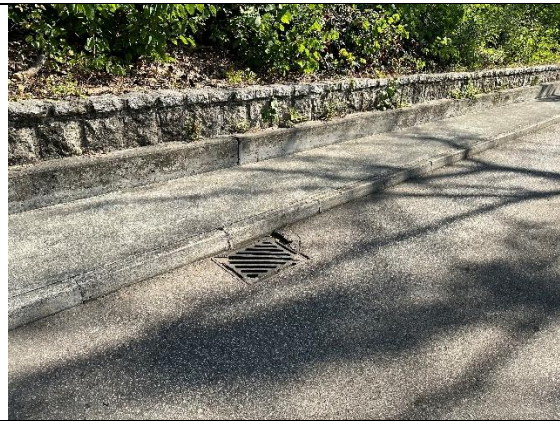
Photo 16 A road gully is located along the road to the north of the Application Site.
