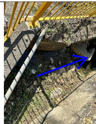
Photo 6 Drainage channel is located along the north side of Fung Kat Heung Road.
