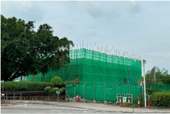
Construction site of Yau Pok Road Light Public Housing
