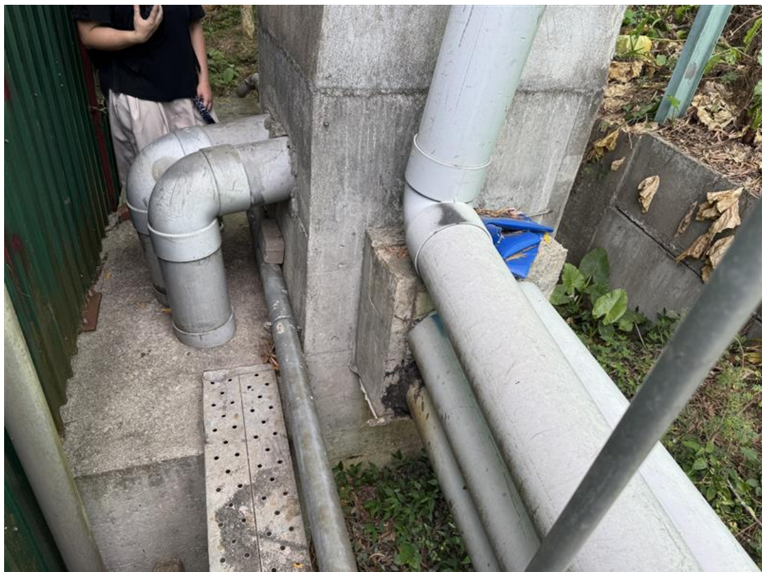
Figure 2: Current inlet of rising mains to Application Site
