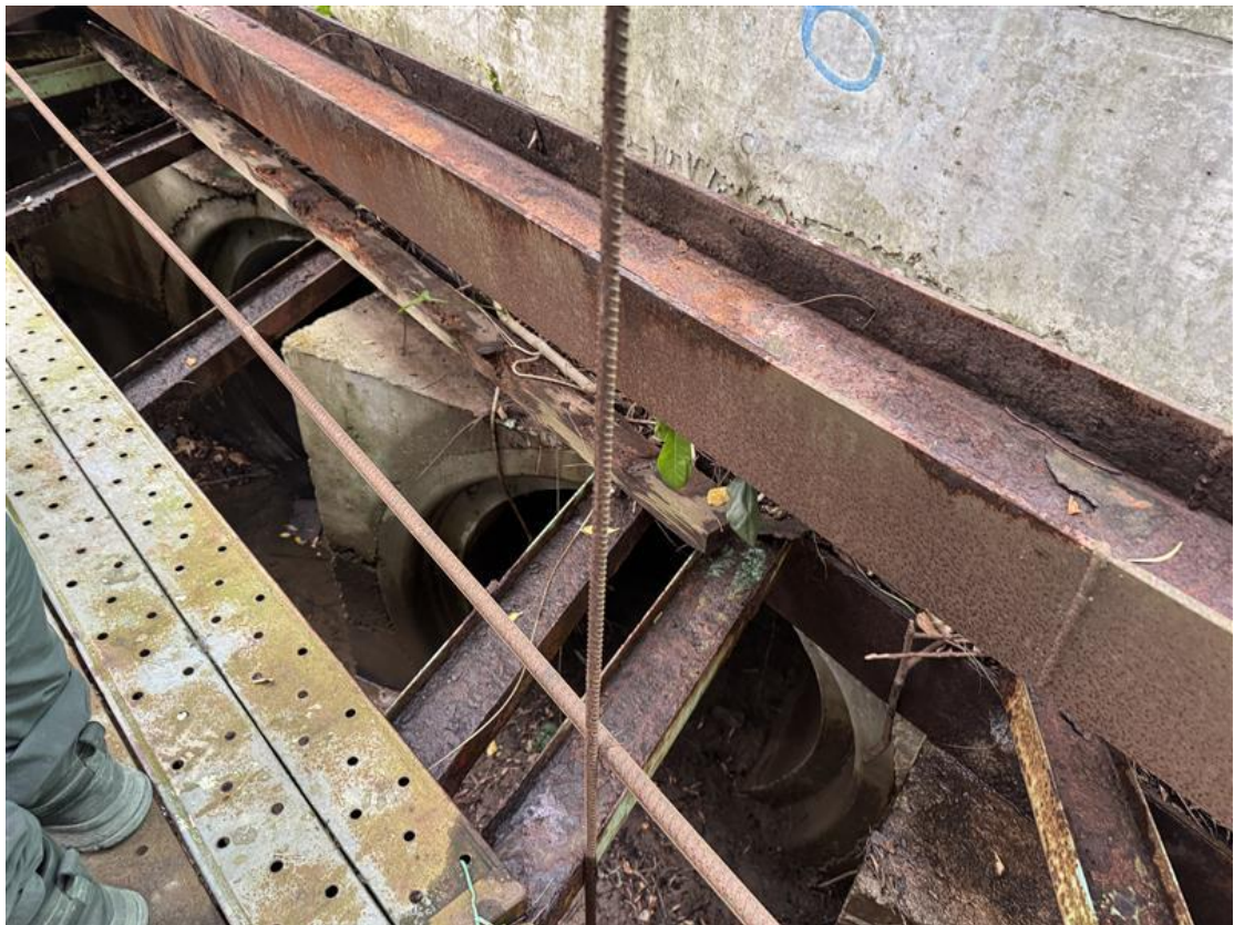
Figure 5: Inlet of triple 1350mm dia. Pipes to east portion of Application Site
