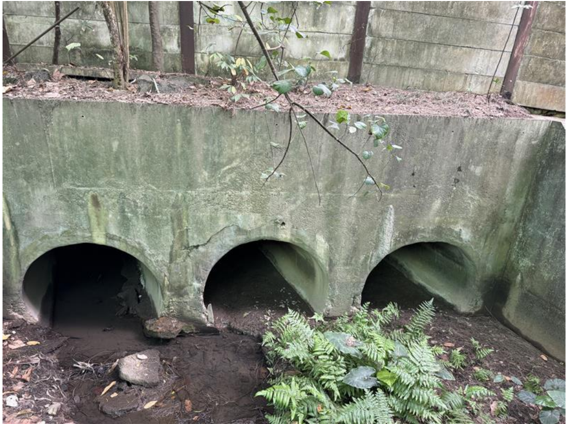
Figure 4: Outlet of triple 1350mm dia. pipes before Application Site
