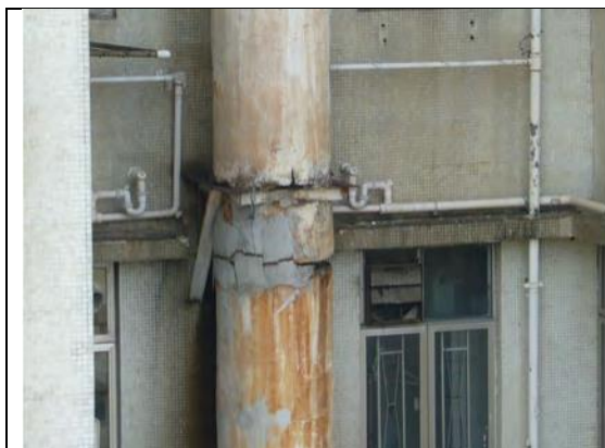
Figure 4.3 Cracks on Chimney Wall in Kwai Fong Terrace
