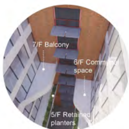
Retained atrium void at Block W
