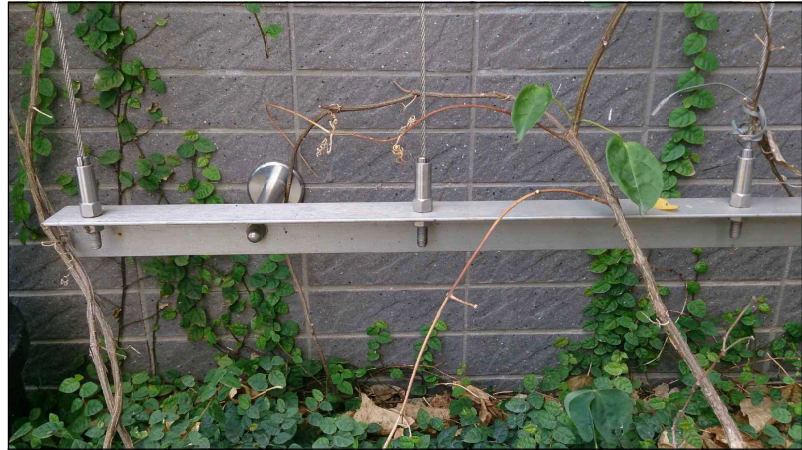
REFERENCE PHOTO OF BOTTOM MOUNTING SECTION WITH EXTERNEAL THREAD END
