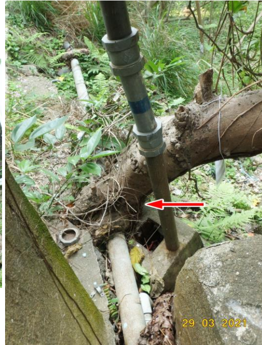
T45 ( Ficus hispida ); Recommendation: Remove Description: Base of T45; embedding nearby pipe.
