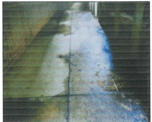
The interior of the water storage house with cracked floor
