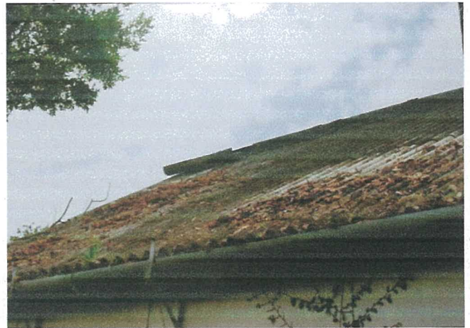
The exterior of the dysfunctional water storage house with cracked roof top covered by Asbestos sheets (photos reported on another local newspaper Apple Daily).
