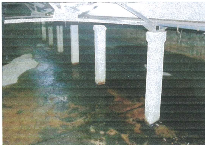
The interior of the water storage house with cracked floor
