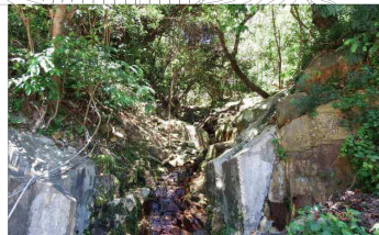
LR2 (B) CHANNELIZED WATERCOURSES FLOWING ACROSS MAN-MADE SLOPE
