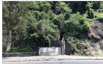
LR2 (E) CHANNELIZED WATERCOURSES FLOWING ACROSS MAN-MADE SLOPE
